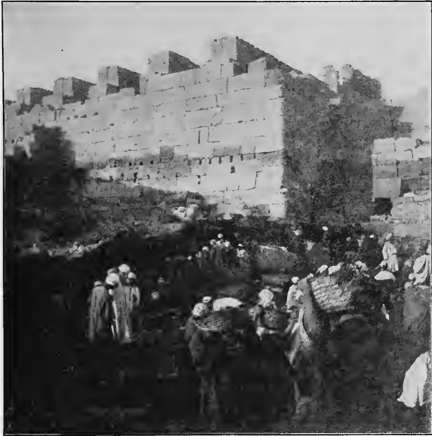
M. LEGRAIN'S EXCAVATION OF THE KARNAK STATUES IN PROGRESS.
